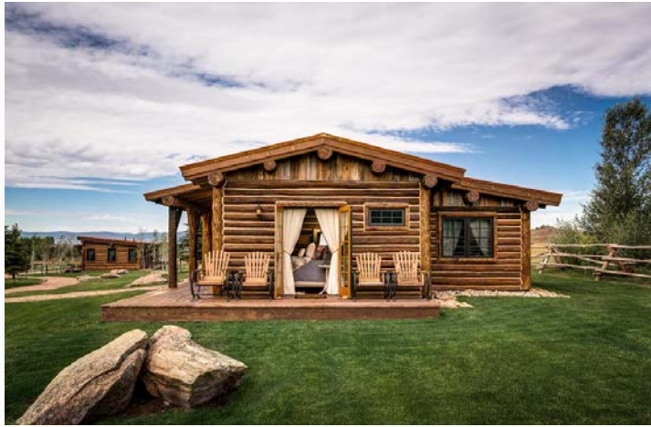
One of the restored log cabins at Magee Homestead / © DAN HAM PHOTO 2012
