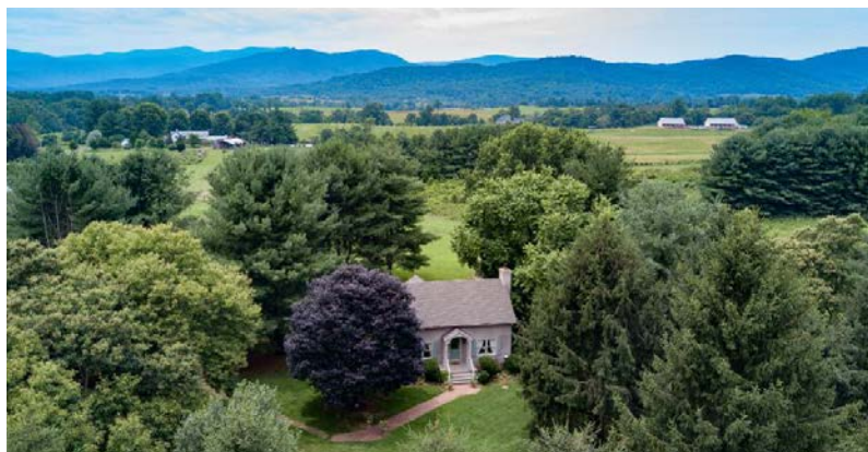
LeFay Cottage at Little Washington / LEFAY COTTAGE
